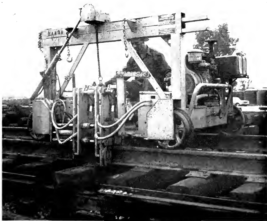
Anchor applicator at work on one of the track-panel jigs.
